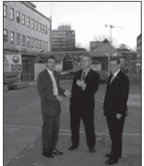
Cllr Peter May on site with Lembit Opik MP and Peter Black AM where demolition has started to make way for the new complex.
